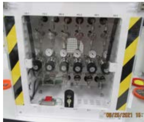
6 Stick GIB for high flow rate process gases
